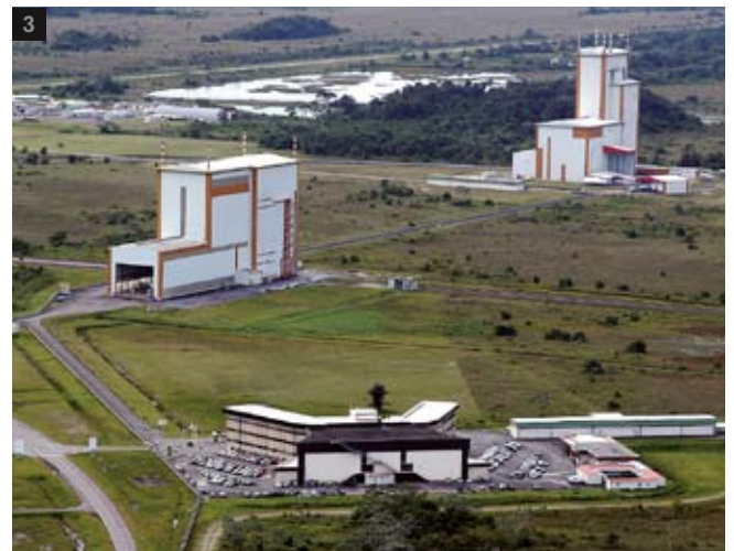
1 & 2 Ariane 5 rocket arriving in ZL3 © CSG/OV P. PIRON, P. BAUDON 3 The armored area of the CDL3 and the BIL and BAF in the background © CSG/OV
